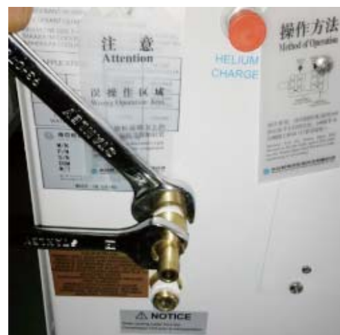
Figure 13 Connect and Remove the Water Lines
